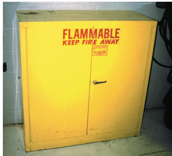
FIGURE 5 Typical fireproof flammable storage cabinet.
